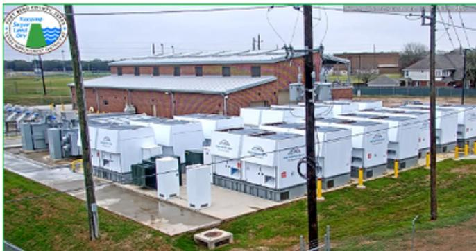
Enchanted Rock 11.2 MW - Fort Bend County LID 2 backup system saved over \$6 million to the district. Since the generators run under load, the system is constantly tested and conditioned, which leads to a higher level of availability than traditional diesel backup.
